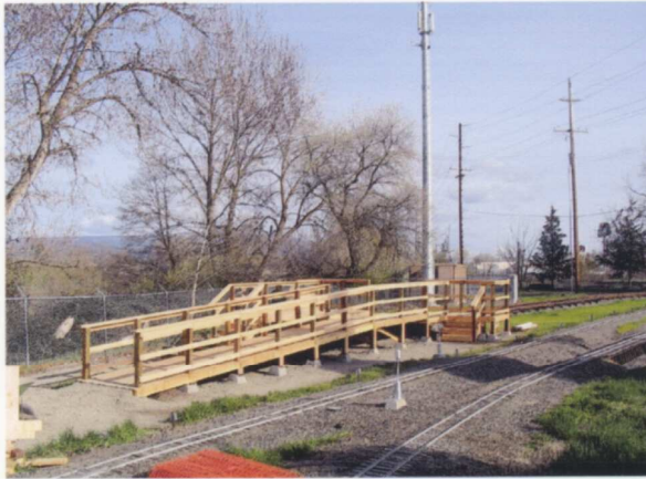
(RIGHT) Last year's temporary loading platform is a memory when compared to the new platform. The public will walk up the wheelchair accessible ramp and be able to board our cars from both sides with ease. Exit staircases on both sides will allow a quick exit and boarding so we can make more trips. — Rick Aubin photo
