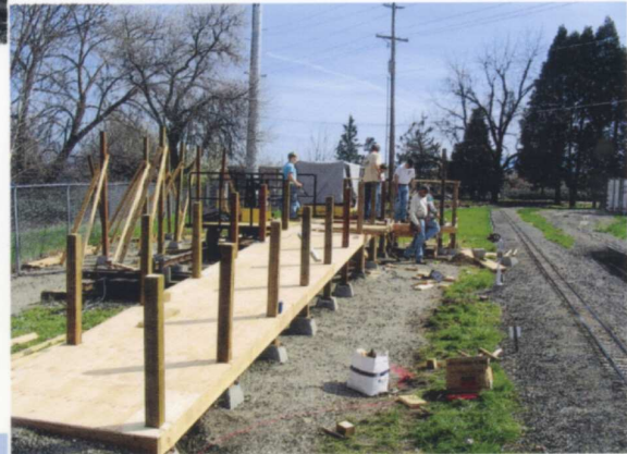
(RIGHT) Last year's temporary loading platform is a memory when compared to the new platform. The public will walk up the wheelchair accessible ramp and be able to board our cars from both sides with ease. Exit staircases on both sides will allow a quick exit and boarding so we can make more trips. — Rick Aubin photo
