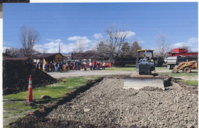
(LEFT) The museum-archive building site had already be scraped and leveled before the day began. Ric did a little bit of earth moving first, then the cameras rolled as a load of shale was dumped on the site. - Ric Aubin photo
