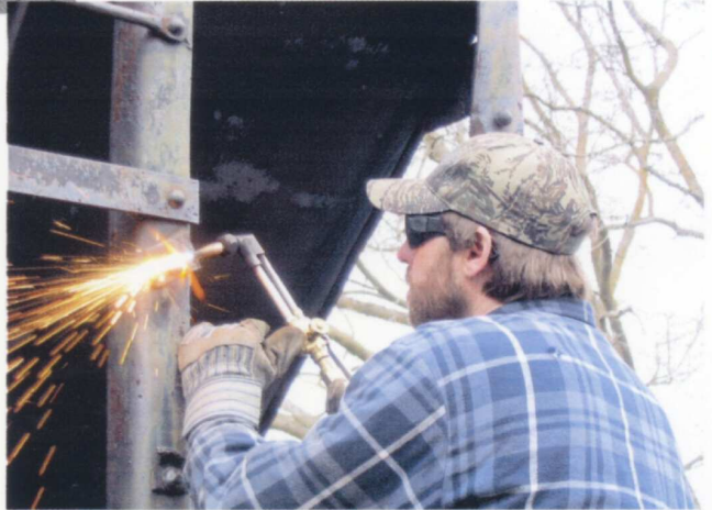
(LEFT) Now it's John Powell's turn to use the torch on one of the rungs. This particular rung only needs a little straightening, so while John heats the rung, Dave applies hammer force from behind. Rick Aubin photo
