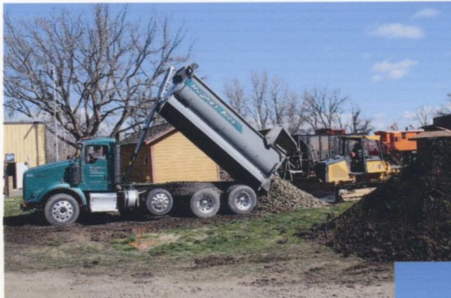
(RIGHT) After the shale was dumped, a bulldozer then quickly spread and leveled the site, and then a load of 3/4 minus rock was laid on top and leveled. Because of the newsletter deadline, next month we'll list the names of all those companies and individuals who donated their time and resources. - Ric Aubin photo
