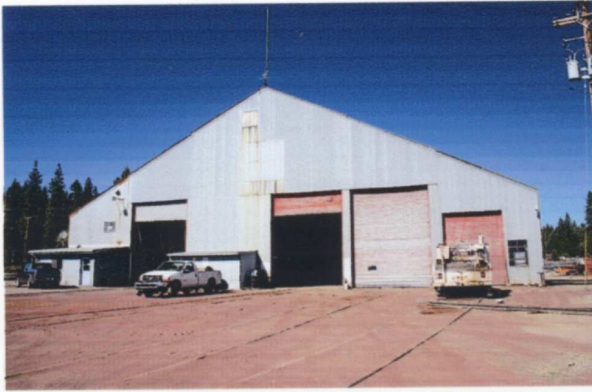
(LEFT) This is the outside of McCloud Railroad's large shop and repair facility in McCloud. Among the equipment inside is McCloud 2-6-2 #25, now up for sale. — Rick Aubin photo
