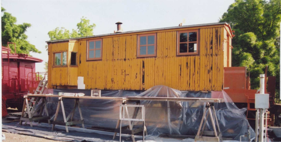
(LEFT) Here's how our SP Flanger looked just prior to repainting. In a few moments Steve will protect the windows from paint with cardboard. At far left is a white test patch of the white paint sealer Steve applied many weeks earlier.
