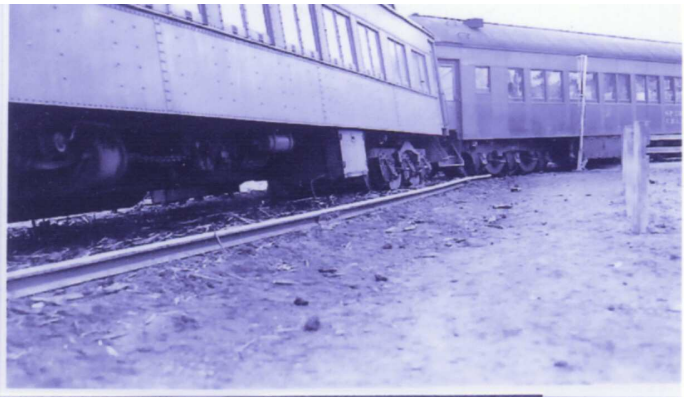
[ABOVE] Daylight has arrived at Selma, and so have most of the town's residents. The photographer is looking south (railroad East) as a large railroad "hook" is re-railing a baggage car. The derailed train did not jackknife nearly as much as some high-speed derailments do.
