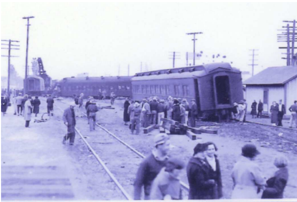
[ABOVE] Daylight has arrived at Selma, and so have most of the town's residents. The photographer is looking south (railroad East) as a large railroad "hook" is re-railing a baggage car. The derailed train did not jackknife nearly as much as some high-speed derailments do.
