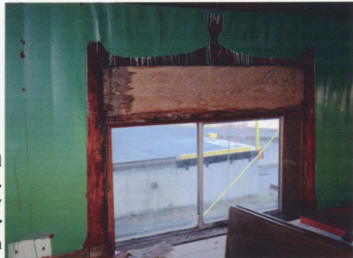
The stained glass was removed long ago and the space above the window boarded over. Then SP painted over the original mahogany with green paint. This was later covered over with cheap paneling. — Dan Wilkinson photo
